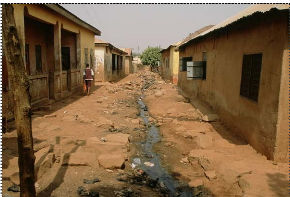
Photo E: A sewage channel running between houses in Woriziehi, Ghana
