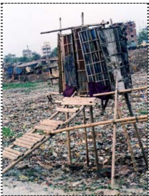
Photo C: A hanging latrine in Dhaka, Bangladesh
